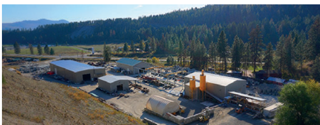
View of the Leko Precast factory in Vernon, British Columbia, Canada
