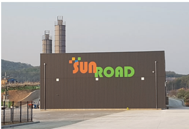
Sunroad's new concrete block plant
