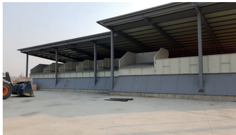
View of the aggregate silos
