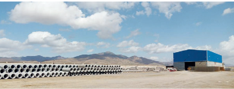
Outdoor storage yard with production hall
