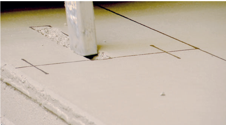
The concrete aspirator removes the concrete which has not cured; it is primarily used to make cut outs for ducts, open cores, hammer heads, protruding reinforcement ends and cleaning of the tracks at the side of the casting bed.
