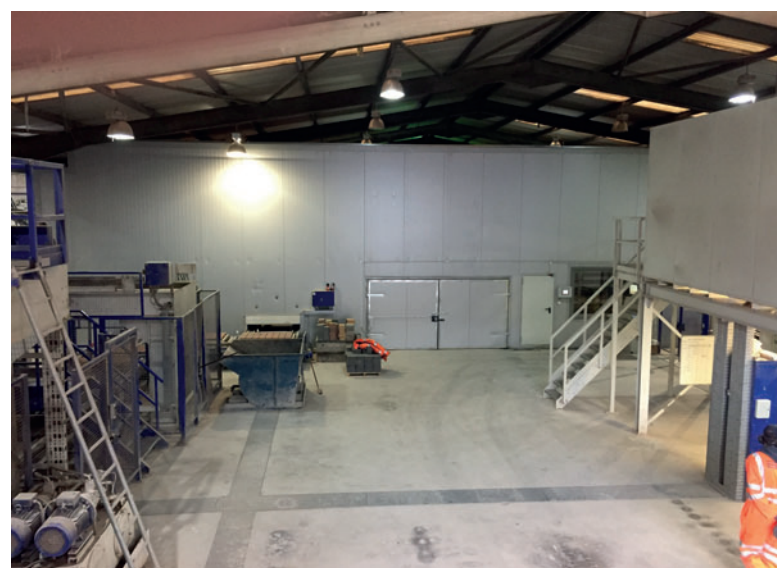
Insulated transfer car area including elevator and lowerator. Double-door for equipment access, personnel door and large window.
