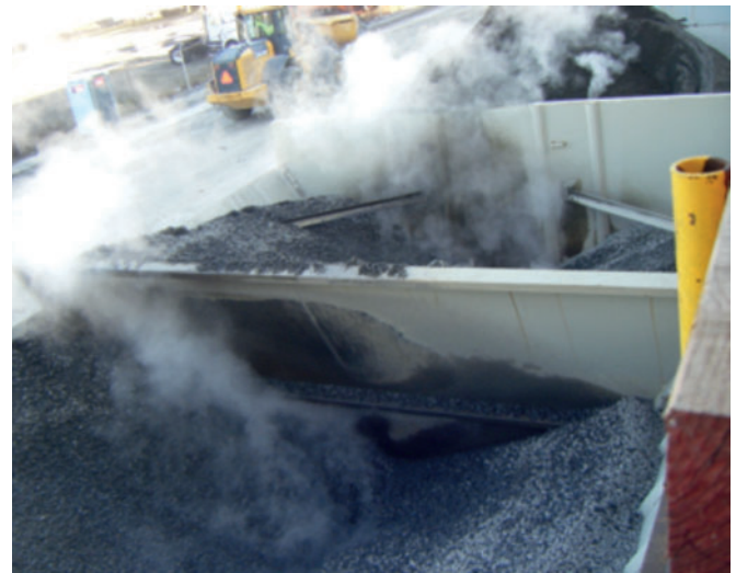
Heating of sand and gravel.
