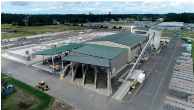
One dump station fills all the bins for both plants and there are supplemental covered aggregate storage areas
