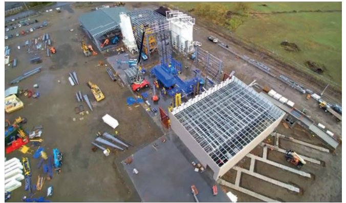
The 105,000 sq. ft. (9700 sq. m) building during construction
