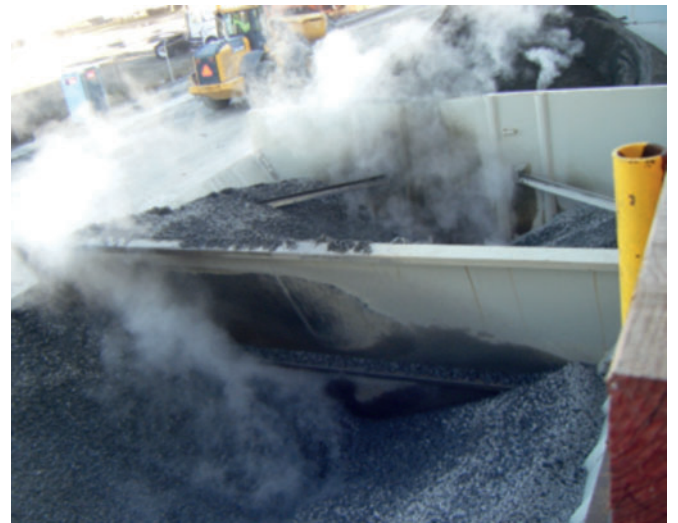
Heating of sand and gravel.
