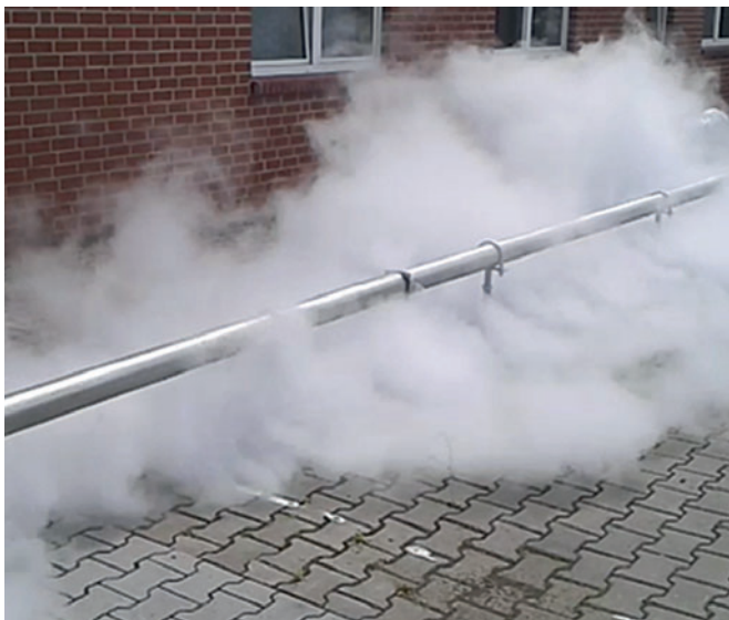
Vapor distribution pipe with holes or a hose connection for the distribution of heat.
