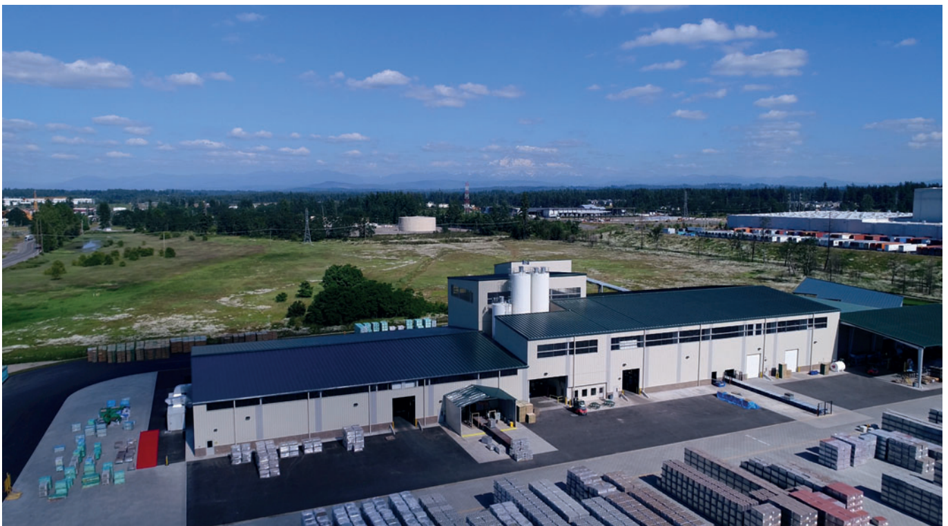
With majestic Mt. Rainier hovering in the background the new plant rises in the foreground
