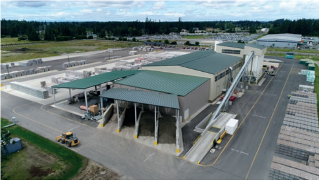
One dump station fills all the bins for both plants and there are supplemental covered aggregate storage areas
