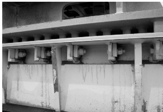
Figure 3: Horizontal bolting
