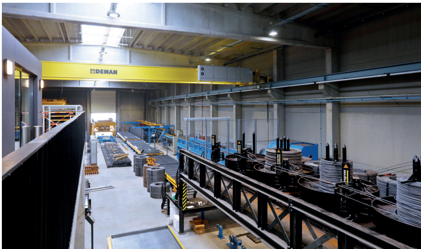
The carrousel system was installed in the smallest possible space and has automated significant individual operations.
