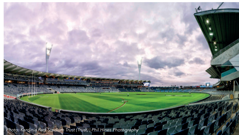
For the Simonds Stadium in Geelong Westkon Precast produced over 8500 m 2 of hollow core slabs and 1250m 2 of the new lower bowl stadium plates.
