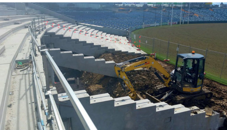
Already, two stadiums have been equipped with the stadium slabs produced by the new slipformer.
