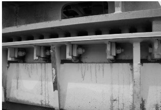
Figure 3: Horizontal bolting
