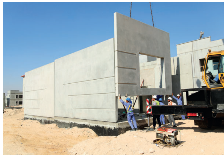
One example of Hi-Tech's precast concrete panels installed in a system for the efficient and quick erection of residential villas, commercial units and mid-rise structures.
