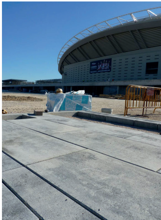
Installation of the concrete blocks used in the outdoor area - photograph
