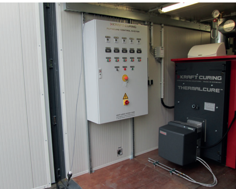
AutoCure Automatic Curing Control System provides for control of casting bed temperature for 6 beds, individually, using threaded temperature sensors, located at the casting beds. An economical and effective curing control system.
