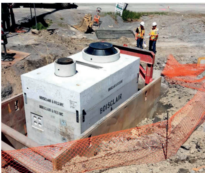
Boisclair et Fils specializes in the production of pre-cast concrete elements for the infrastructure sector, both for water and wastewater, and the electricity and telecommunications branches.
