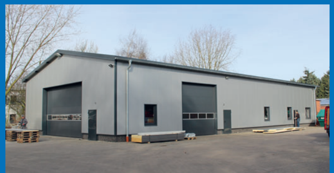
Kraft Curing Systems GmbH headquarters in Lindern has been extended by a new 450 m 2 hall.
