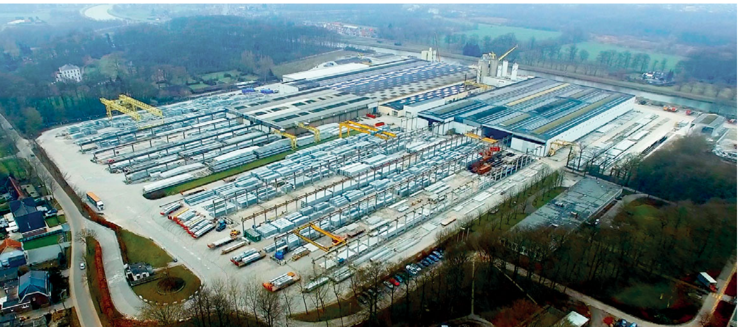
Factory grounds totalling 49,000 m 2 structural precast concrete elements, wall elements and hollow core slabs are produced. The total works site of the company, founded in 1963, covers a surface of 240,000 m 2 .
