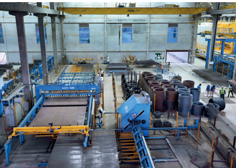
Thanks to their efficiency the three systems installed for the manufacture of reinforcement (the picture shows the mesh welding plant) contribute to optimum production continuity.
