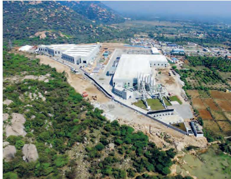
In the KEF Infra One Park near Bangalore the majority of that which is required for the construction of residential and commercial buildings is being produced.
