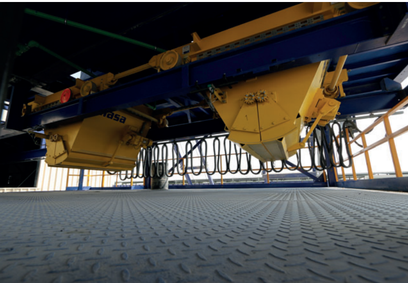
The ready mixed concrete will be transported to the block making machine by a double bucket conveyor
