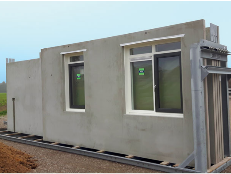
Geelen Beton's declared goal is to shorten the construction time. For instance, the windows are already pre-installed in the plant.
