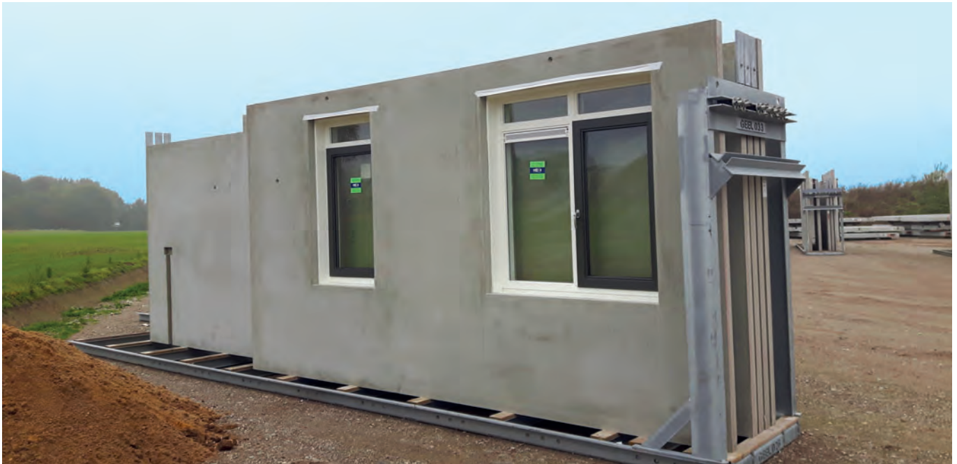
Geelen Beton's declared goal is to shorten the construction time. For instance, the windows are already pre-installed in the plant.
