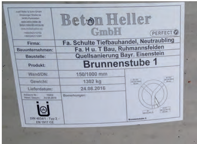
A label on the finished, cast water chamber providing information on all the relevant product parameters and project data.
