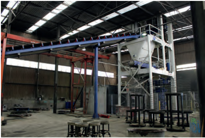
Concrete feeding to the RP 1630
