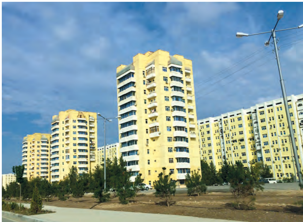
Affordable and modern living space is to be created with the aid of state programmes. Precast technology is playing a big part in this project.
