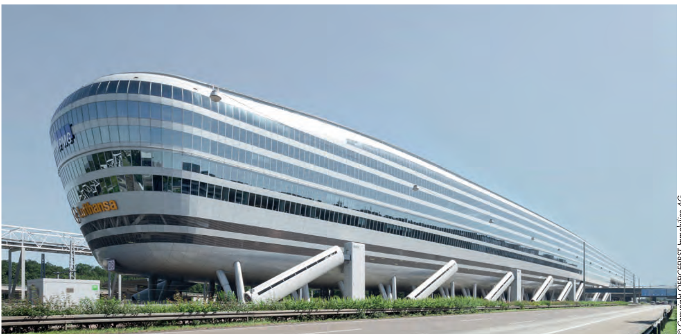
In order to guarantee optimum customer support, part of PSD was located in the Progress Group office in "The Squire" at Frankfurt Airport. Customers not just in Germany, but all over the world can thus be reached easily and quickly.
