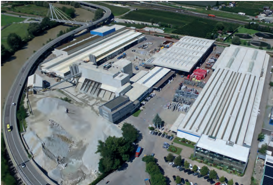
The PSD development team elaborates software solutions for the reinforcement and precast industries in Brixen (picture shows the headquarters with its own precast plant) and in Frankfurt am Main.
