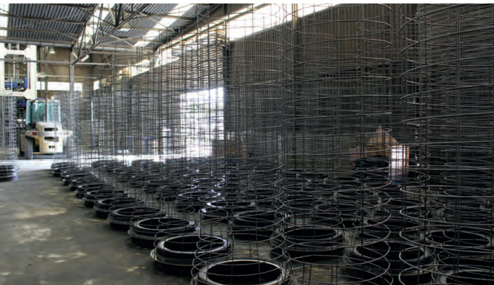
Base pallets with reinforcement stand at the ready
