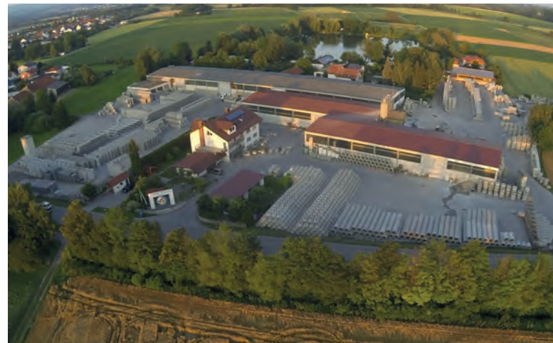
Production of high quality precast concrete components for the underground construction market has been ongoing at the Josef Heller & Sohn GmbH site in Parkstetten, Straubing, for over 60 years.
