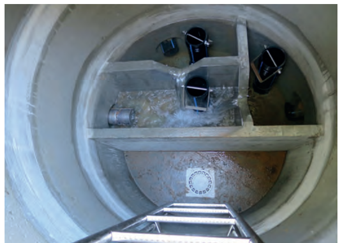
View inside a DN1500 concrete water chamber tailor-made by Wyss AG, with multiple inlets and 4 chambers at the water catchment site in the municipality of Vitznau, on Lake Lucerne.
