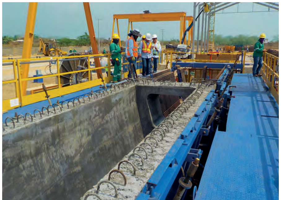
A vibration and heating system ensures steady compaction and curing of the concrete used. V girders in three different lengths, weighing up to 85 t, were produced for the "viaducto Gran Manglar", the longest road bridge in Colombia.
