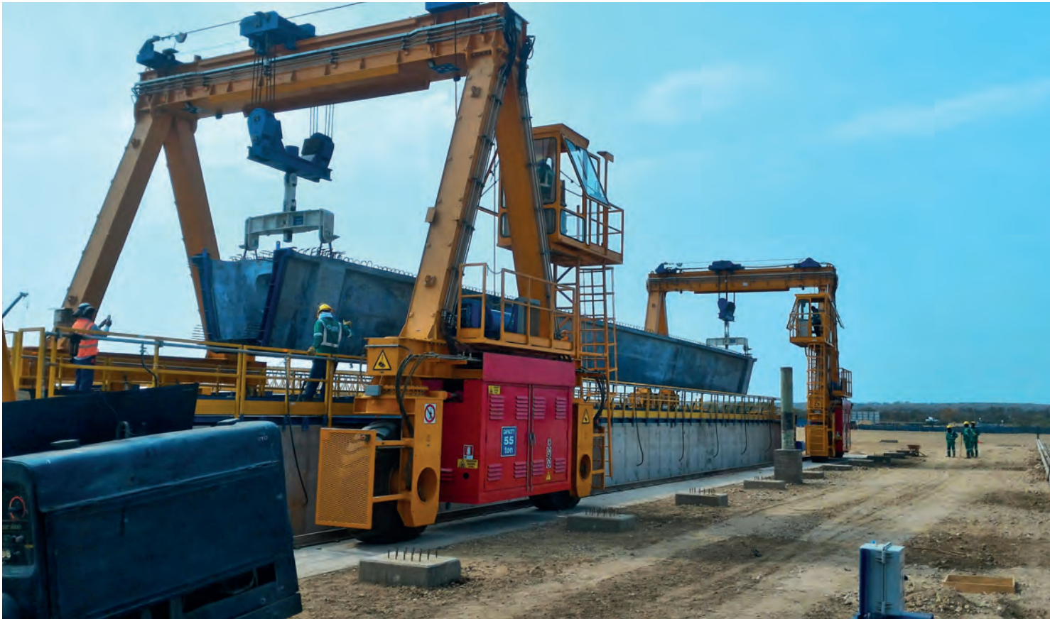
Two gantry cranes load a total of 387 concrete elements on to special HGVs, which transport them to the construction site.
