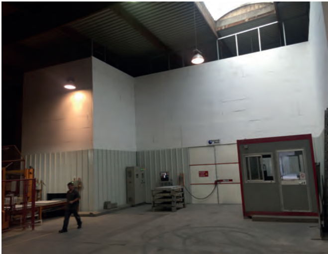
Enclosure of the transfer table aisle and the elevator and the lowerator ensure an energy-efficient system and protect the finger car.
