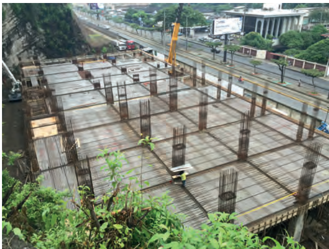
In August this year a five-storey car park was constructed for the Catholic University of Guayaquil. An addition of two more levels is planned.
