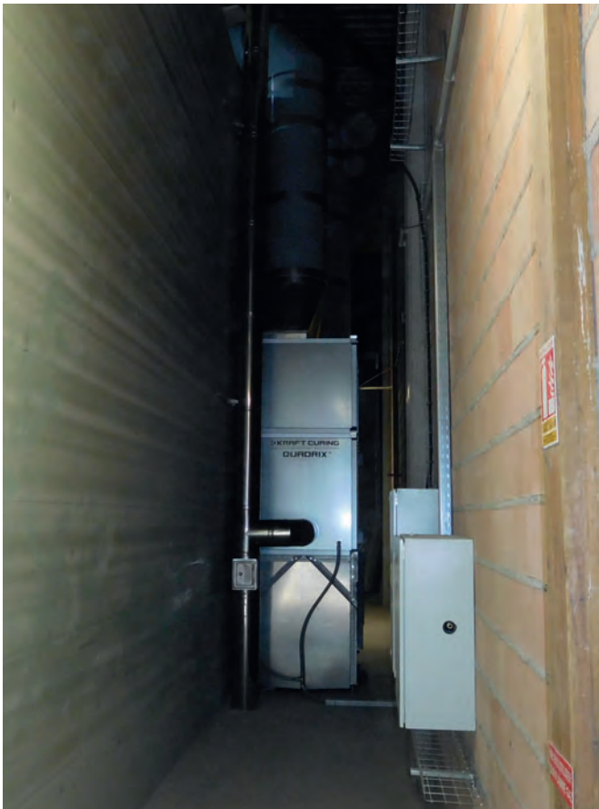
The Quadrix® circulation and heating unit stands behind the chamber and takes up little space. The control cabinet and humidifying system stand nearby.
