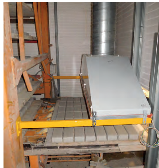
One of two heated hoods installed between the lowerator and chamber wall prevent the escape of warm and moist air, preventing any condensed drops of water reaching the fresh blocks.
