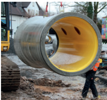
Lifting of a ready-to-install Perfect Pipe with two lateral inlet openings.
