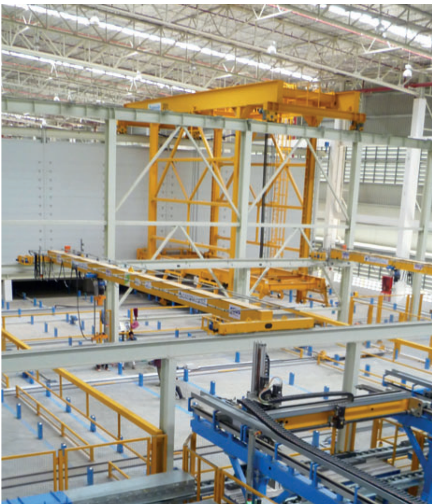
The pallets are put into and taken out of storage by a fully automatic storage and retrieval machine. ebos® calculates the necessary dwell time in the hardening rack and transmits this data accordingly to the machine.
