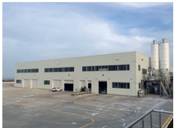
The new production facility halls were erected in a very short time according to specifications from Prinzing-Pfeiffer
