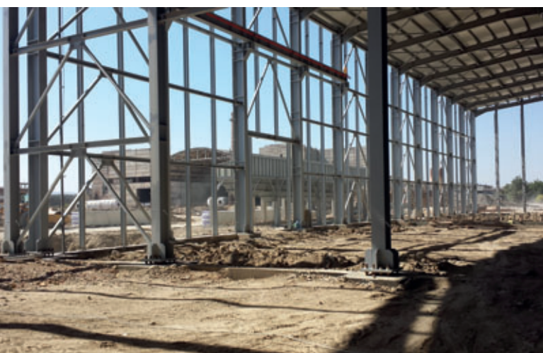
The first production halls standing only 10 weeks after beginning construction
