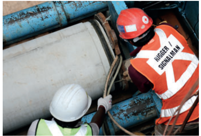
Preparation of the jacking devices
