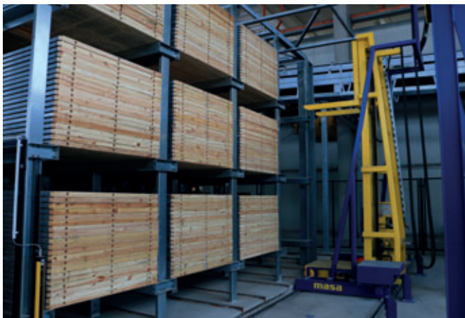
A pallet transporter takes full stacks and brings them automatically back to the concrete block making machine or else places the stack in an intermediate storage rack
