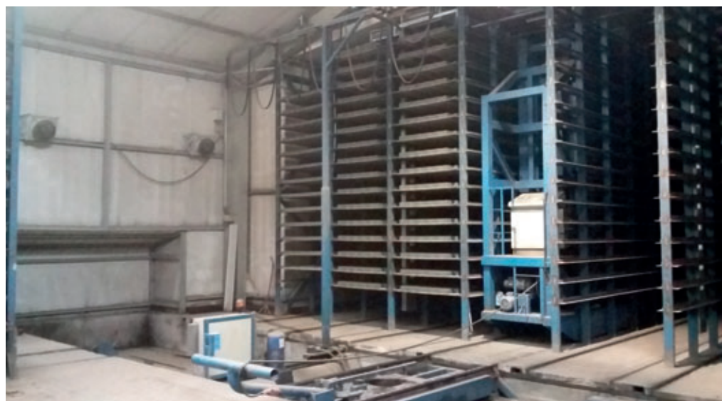
Thanks to the circulation of air in the transfer car area, both this area and the transfer car remain dry. No condensed water forms on the ceiling and there is no mist formation, which could lead to failure of the finger car's laser distance measuring system.
