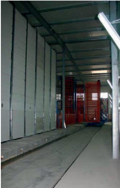
2001 – Transfer Area with 11 individual curing chambers and insulated doors
