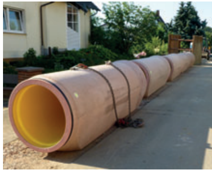
In the first project in the German state of Hesse, Perfect Pipe is being used in nominal width DN800.
