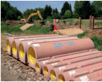
Different pipe and shaft components of various nominal widths, manufactured using the Perfect process.
