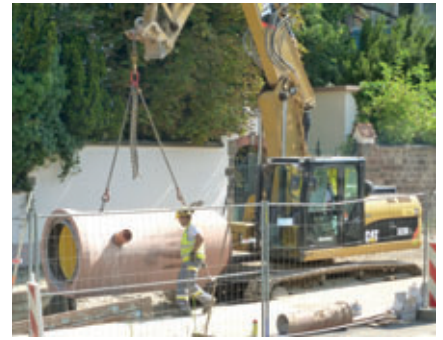
Multiple old ceramic pipelines are replaced by a new DN1000 collector.
