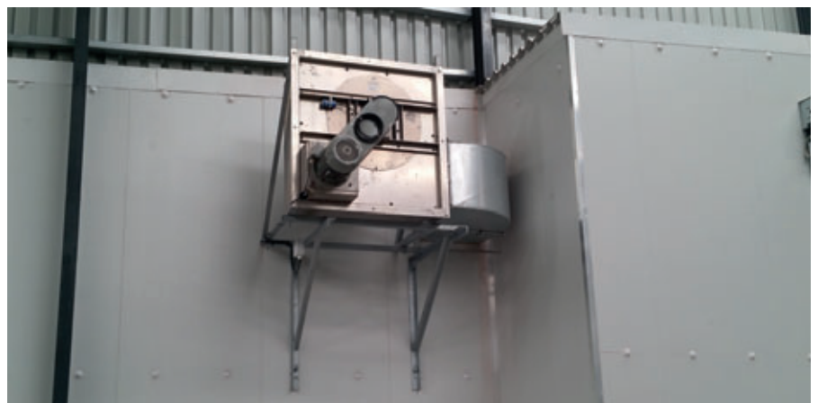
Nautilus Radial Air Circulation Ventilator, manufactured exclusively by Kraft Curing of stainless steel and aluminum in order to provide a durable and effective solution for consistent air circulation in a single atmosphere curing chamber.
