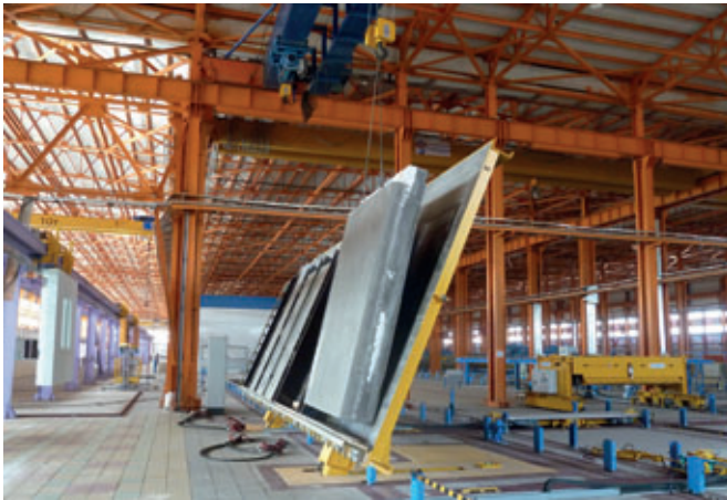
Raising the finished sandwich wall with the help of the tilting mechanism.
