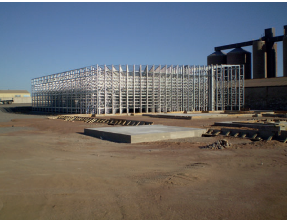
Curing rack galvanized steel erection completed.
