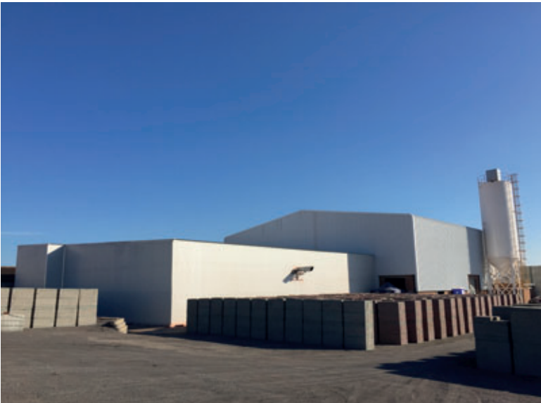
Completed factory with exterior curing chamber (lower building).
