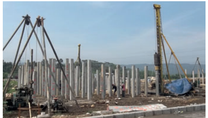
Stabilization of the building soil by using concrete piles.
