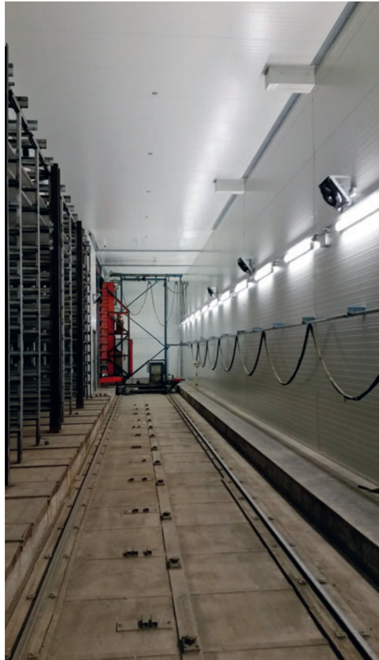
After: insulated walls and ceiling, air circulation & lighting
