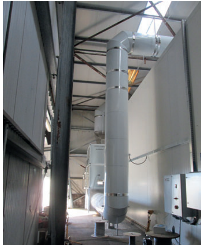
After: stainless steel finished and insulated air heating unit with aluminum frame - 50% less heating capacity than previous model. GFK (glass fibre coated - inside and outside walls) duct with 50 mm Polyiso insulation. Tongue and groove construction with stainless steel compression bands at all joints. Insulation panels on chamber walls and ceiling tongue and groove design with sealed u-channel at the floor and insulated and sealed joints.
