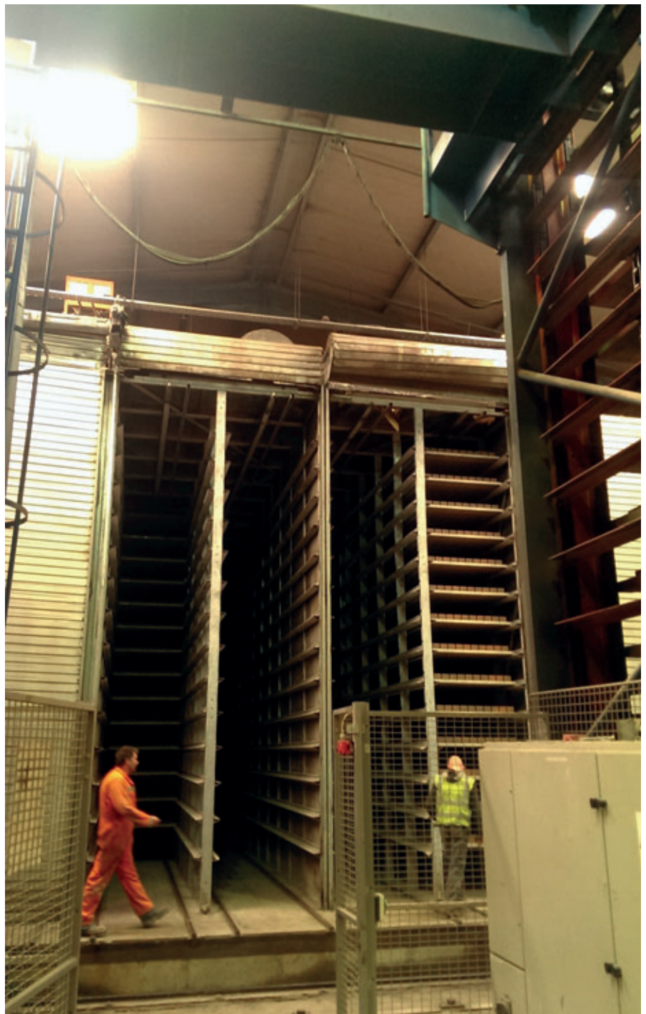
Before: picture of transfer car area taken from beside the elevator
